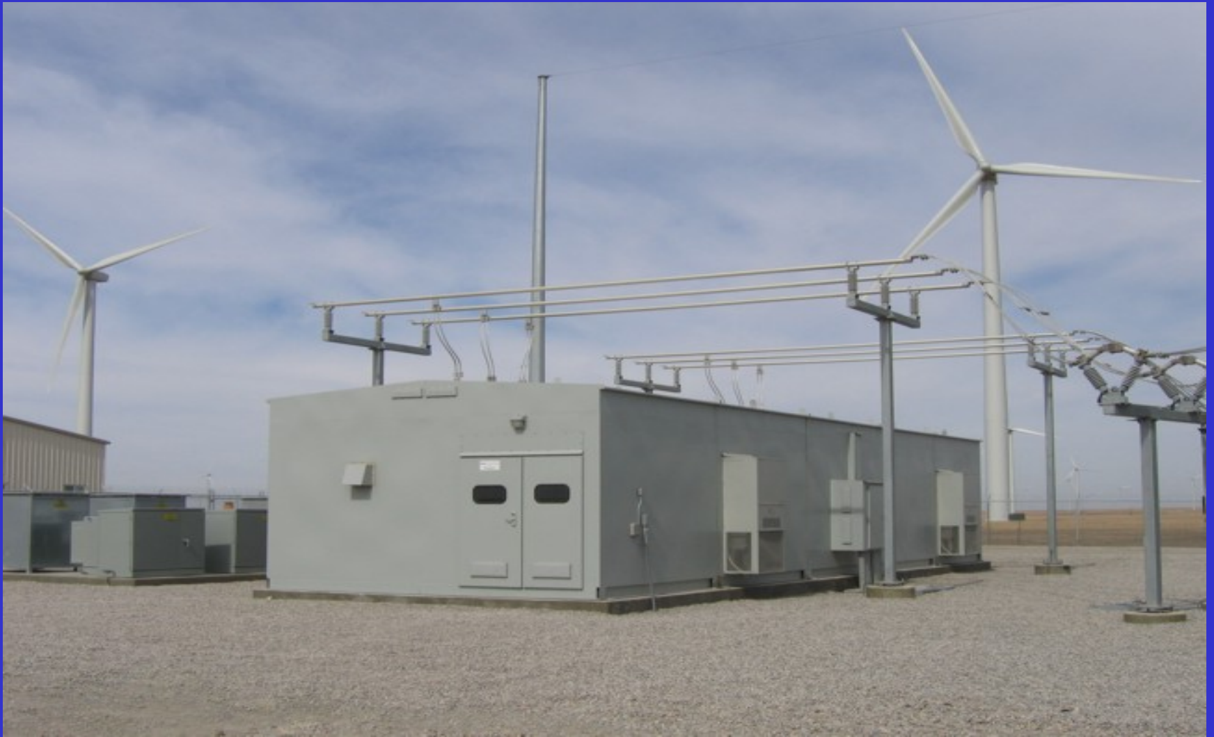
38kV MetalClad Switchgear For Windfarm
