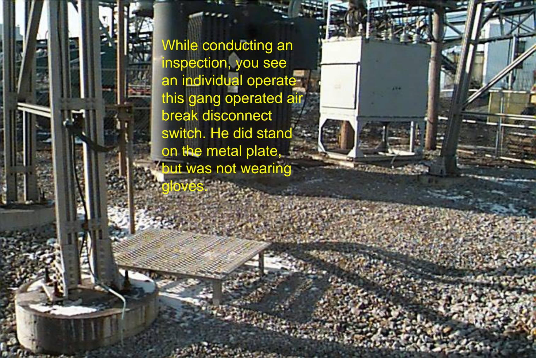
A photograph of an electrical substation. In the foreground, there is a metal platform with a grid pattern on a gravel surface. To the left, a vertical metal structure supports a gang-operated air break disconnect switch. In the background, there is a large white metal cabinet on a metal frame, surrounded by other electrical equipment and metal structures. The ground is covered in gravel.
